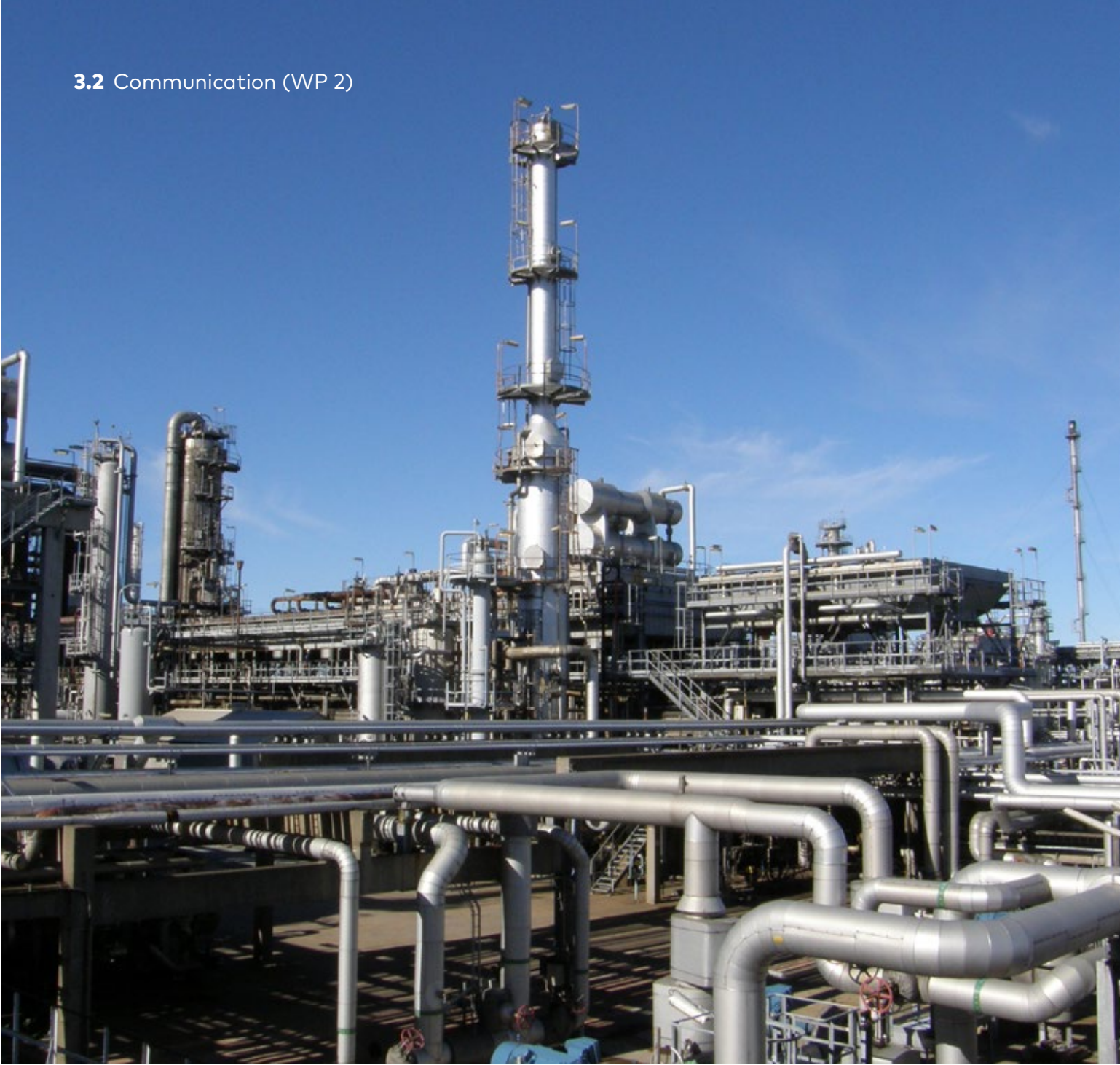
Preem Refineries, Sweden. Photo: Preemraff
