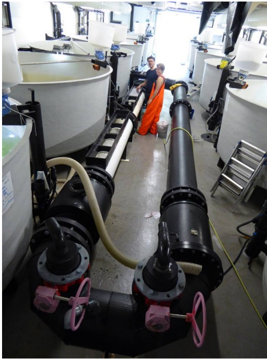
Figure 17 A large swim tunnel system for swimming of large individual fish and fish groups.
