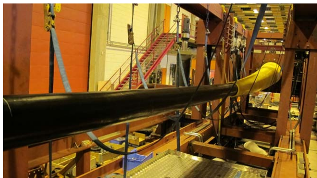
Figure 2. Power cable (black) and bend stiffener (yellow) installed in the rig.
