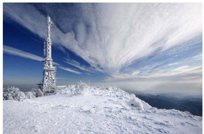
Icing on antennas degrades the total performance on navigation and communication systems. (Photo: Shutterstock)
