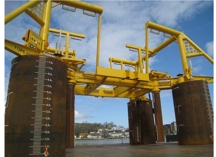
A four-slot integrated template structure for use on the Norwegian Continental Shelf. (Pribytkov, 2017)
