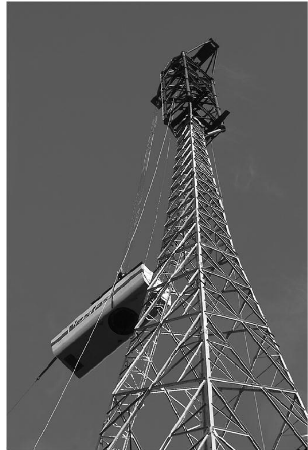
Figure 18.14. Assembly of a Vestas V-66 on a 117-m-high lattice tower, using a top crane extension
