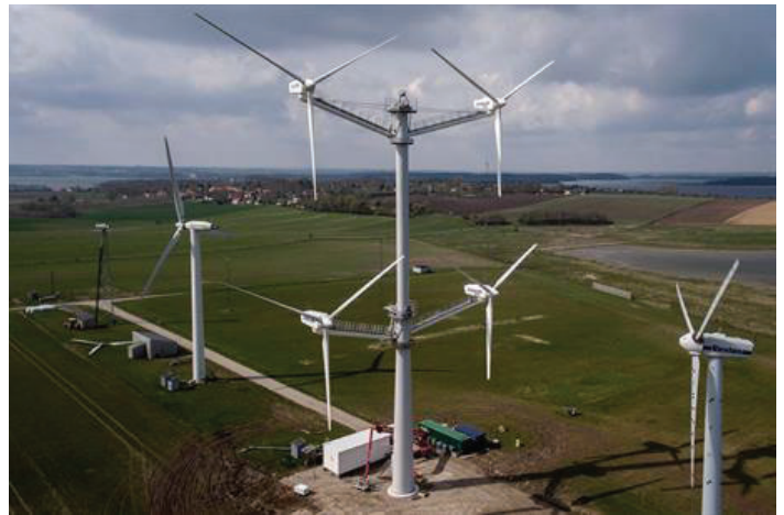
Figure 2: Vestas MRT demonstrator situated at Risø DTU in Roskilde Denmark. Image courtesy of Vestas Wind Systems A/S [2].
