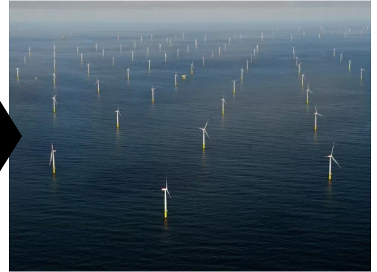
Hornsea Project 2 (165 WT, 1386MW, 2022)
