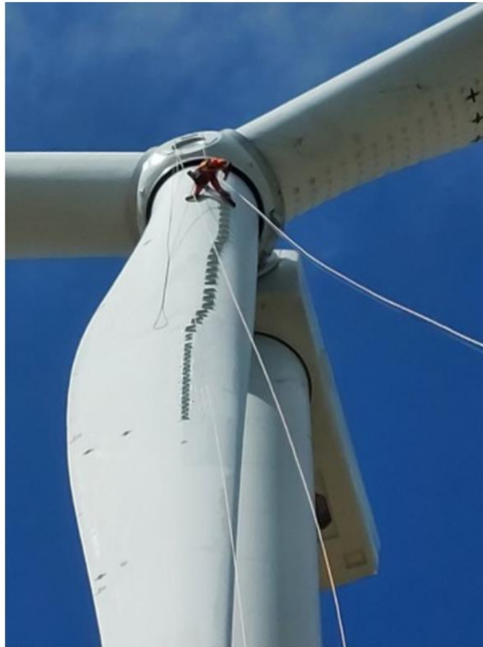
(a) Installation of VGs using rope access
