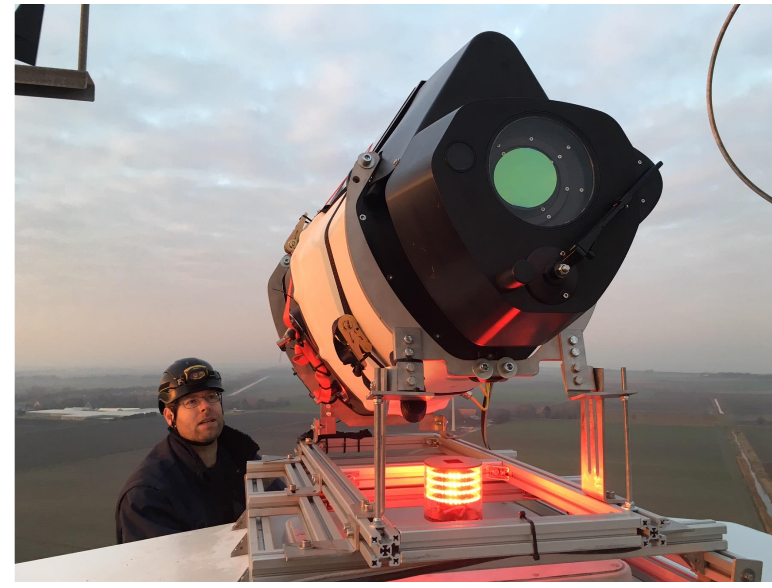
Nacelle LiDAR installation
