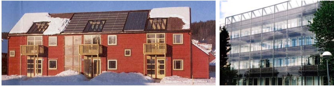
Figure 3-5 PV-modules integrated into the roof construction of two storey undetached houses at Hamar, Norway (left) and into the combined thermal/PV “BP-double skin facade”, NTNU, Gløshaugen (right).
