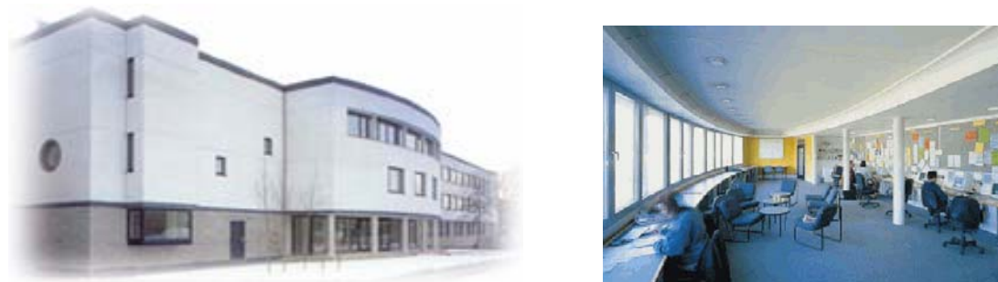
Figure 3-3 The main entrance of the Elisabeth Fry building (left). An IT resource room is located directly above the main entrance, and follows the gentle curve of the elevation (right). Note the row of annular soffit diffusers connecting directly to the exposed TermoDeck slabs.
