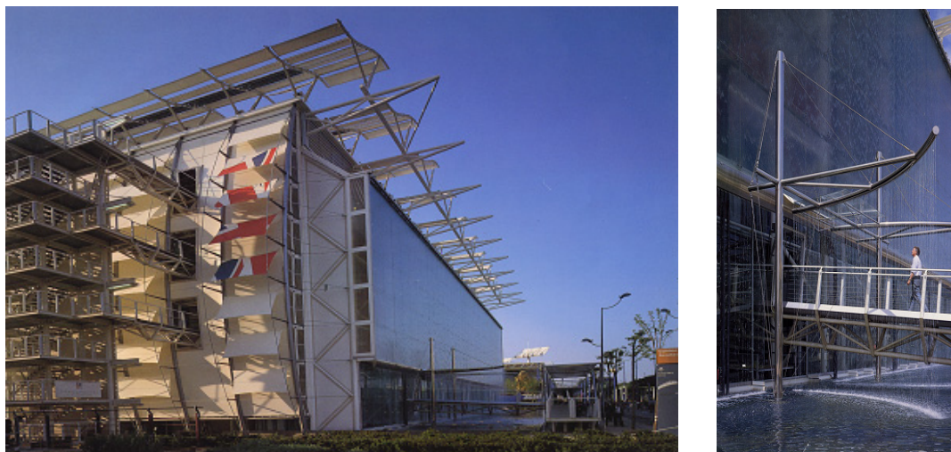
Figure 2-9 British Pavilion, Expo 92, Seville, Spain (architect Nicolas Grimshaw)(left). The east facing “water-wall” (right). The surface evaporation of water limit the maximum glass temperature to around 24 0 C, and thus provide cooler internal environment. In addition, the curved shadings on the roof shields it from sun and limits the rise of internal temperature.
